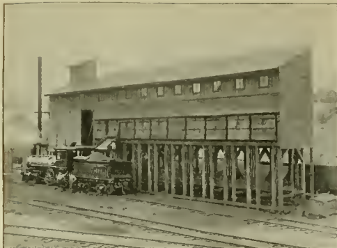
Fig. 1. Front View of Coaling Station.
